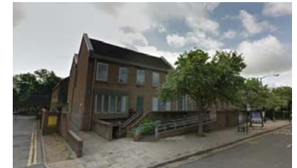
Existing RBWM office, York House, Sheet Street from north
