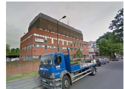
Existing TVP office, Alma Road, from south
