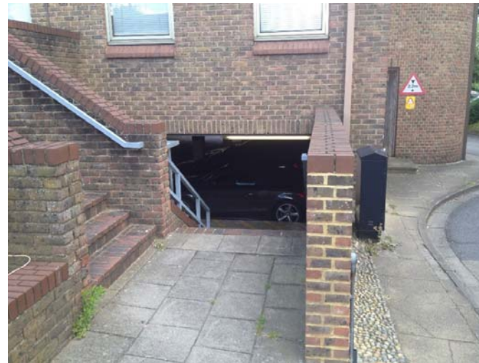
Level change from Sheet Street into undercroft car park
