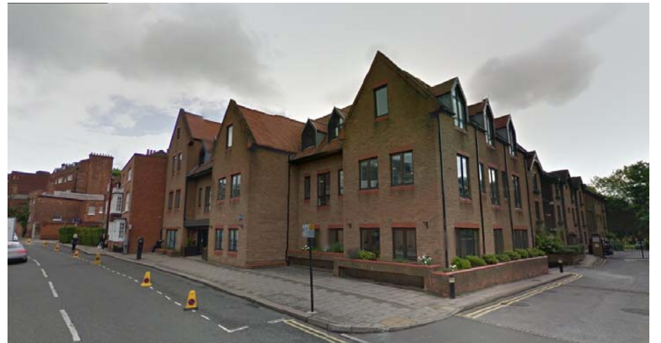
Parkside House to the north of the site
