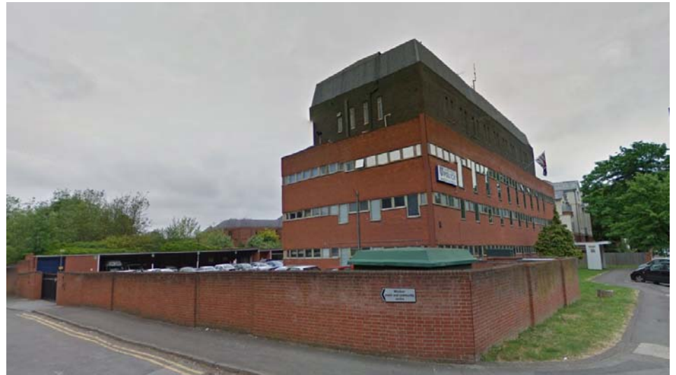
Boundary wall on the corner of Alma Road with refuse storage behind
