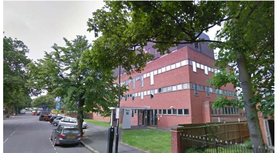
Existing Police Station and frontage parking
