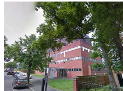
Existing TVP office, Alma Road, from north
